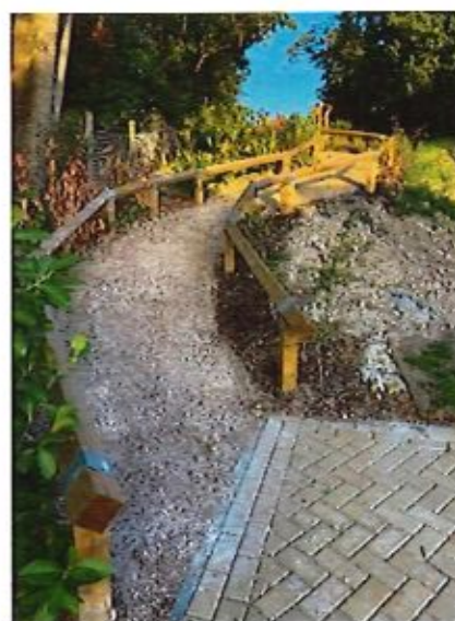
Narrow, steep hoggin footpath leading to stepped railway bridge crossing
